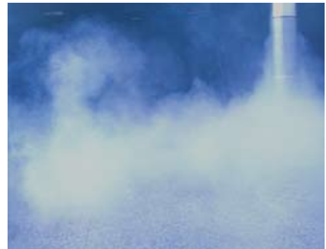
Displacement diffuser type QR-KH - 2000 dia. 580 for heating applications V_{supply} = 5000 \text{ m}^3/\text{h} \Delta T = -5K
